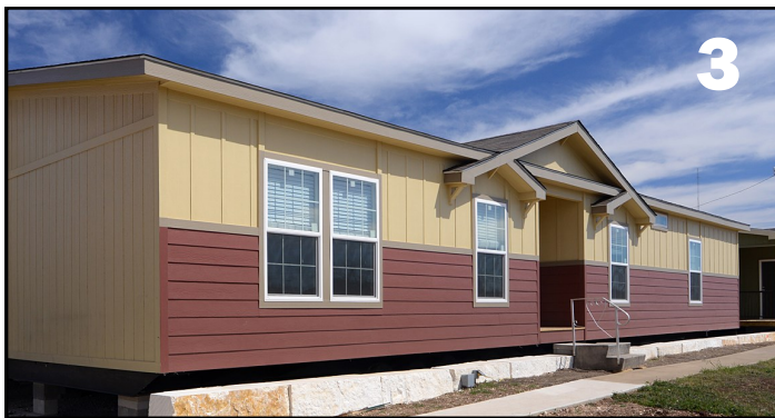
3 Board and Batt with 8 rows of lap at the bottom (choose between lap rows on front or whole house)
