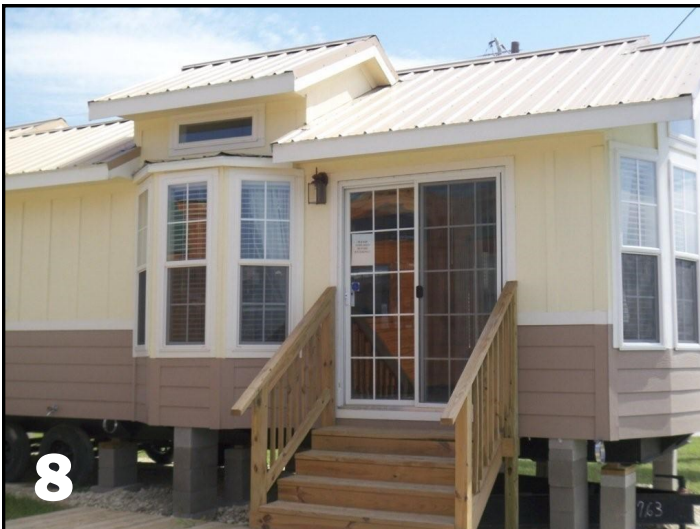
Estate Exterior (board and batt with 5 rows o lap at the bottom and a trim colors on eaves, above lap and around windows and doors)
