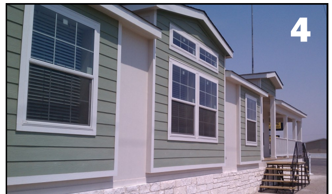
4 Board (no Batt) with bump out box bays and tower dormer with lap inside them
